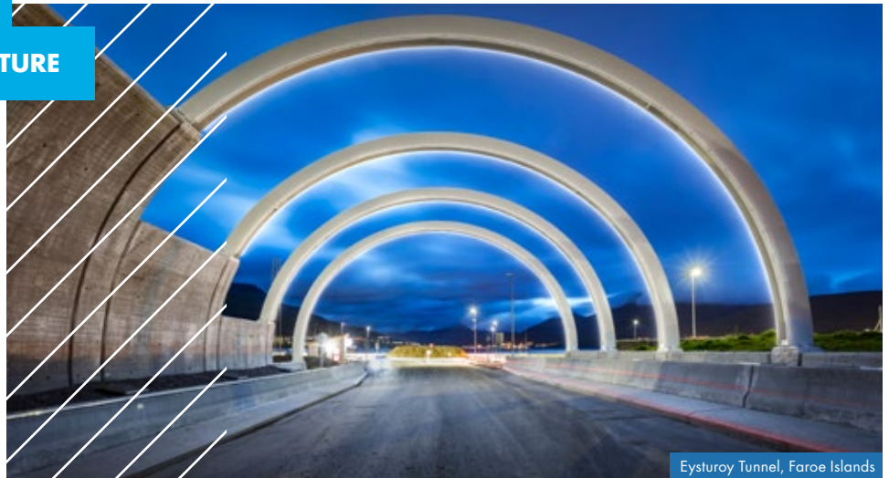
Eysturoy Tunnel, Faroe Islands
